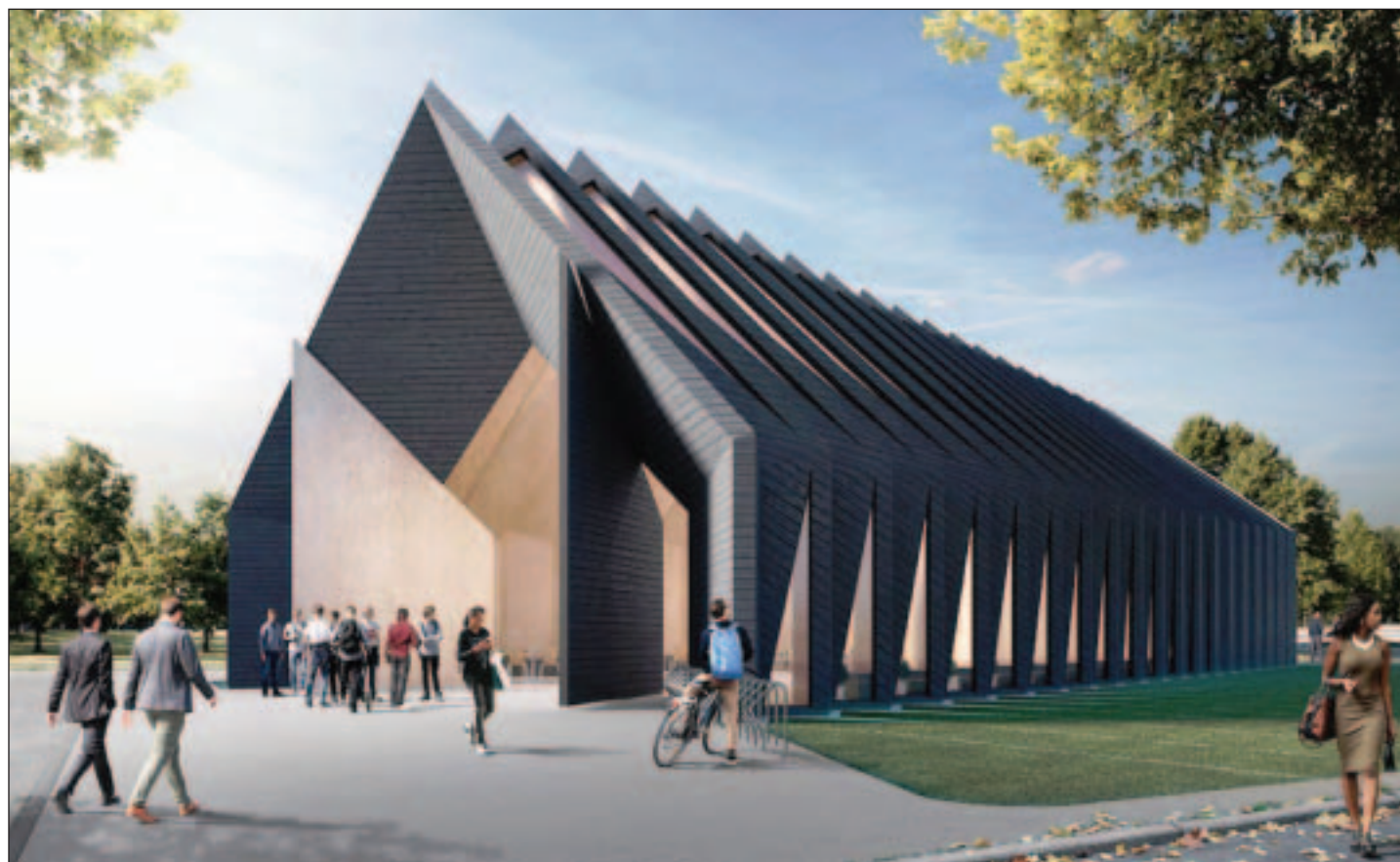
An architecture class at the Massachusetts Institute of Technology (MIT) has designed a longhouse made primarily of laminated veneer lumber. Image: MIT
